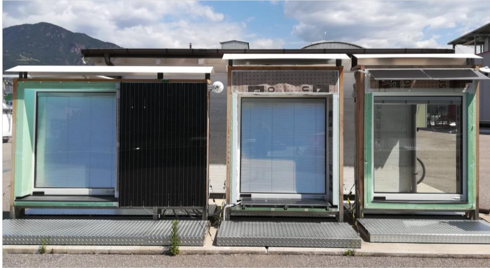
Fig. 1: Solar Window Block mock-ups in the outdoor lab (from left to right: BIPV vertical, BIPV sill, BIPV overhang)
