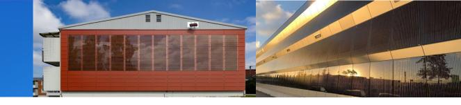
A novel way for fast and easy installation of BIPV modules with the Click&Go solution: The PV panels can be installed by a single person and it can be used in every wind zone up to a height of 200 metres.
